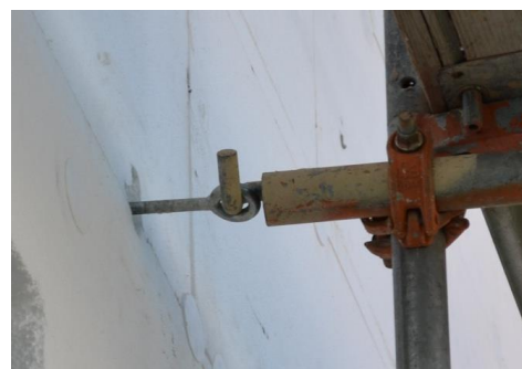
Figure 2. The fixing of an anchor to the insulated façade.
