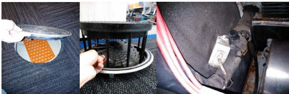
Figure 6. Walkthrough inspection shows improper underfloor diffusers and malfunctioning valve actuator.
