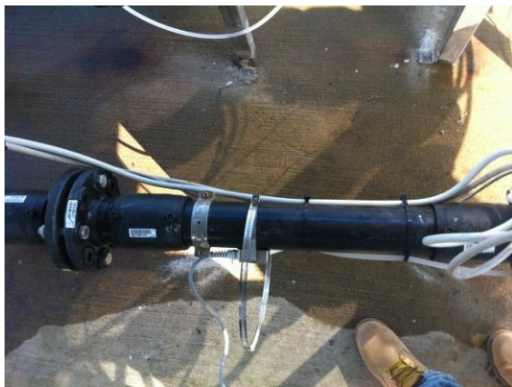
Figure 10. Ultrasonic Doppler sensor installed in the water cabin pumping in Portoverde Marina.
