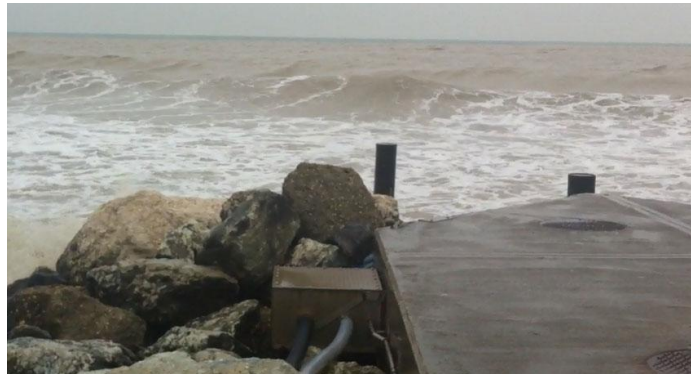
Figure 13. Metallic box installed near the dock and connected with discharge pipes of the ejectors.
