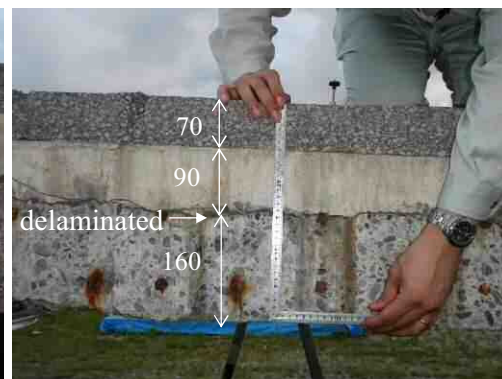
Picture 4. Overlaid area (delamination)
