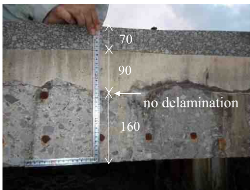
Picture 3. Overlaid area (no delamination)
