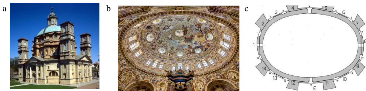
Figure 1. (a) Regina Montis Regalis Basilica; (b) The Basilica dome; (c) The strengthening system installed in 1987.
