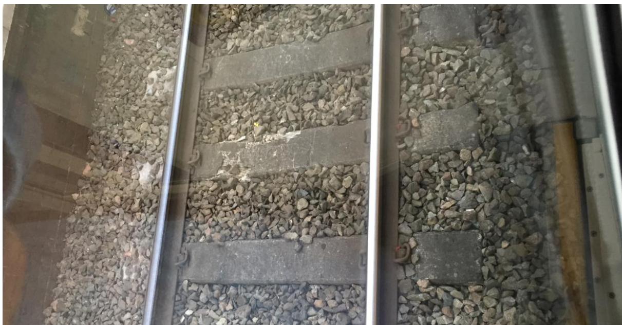
Figure 7. Broken concrete sleepers (taken from a vibration-sensitive track between Solihull and Birmingham).
