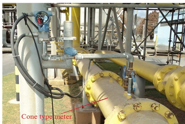
Figure 4. Measuring system of the industry with a cone type flowmeter.
