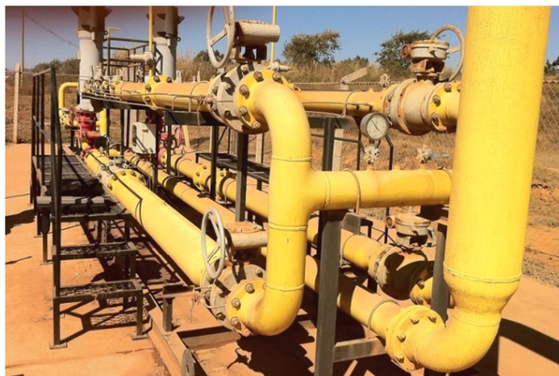
Figure 3. The gas distributor measurement system with turbine meter.
