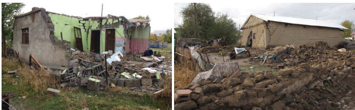
Figure 12. Improper mortar use such as mud
