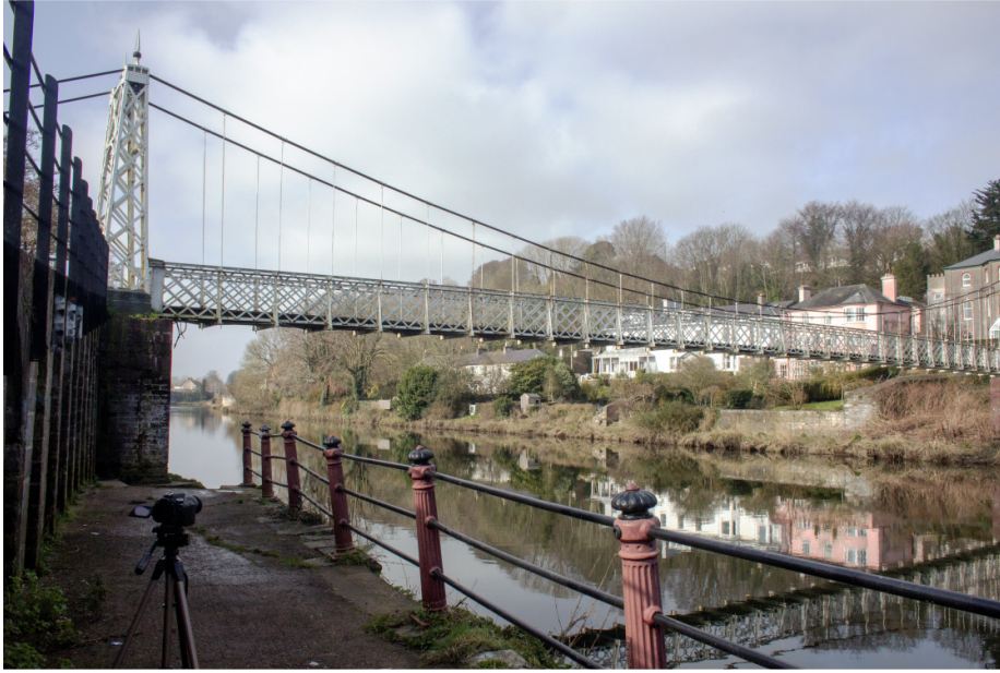
Figure 1. Daly's Suspension Bridge in Cork, Ireland, and the location of a mounted video camera on the river bank.
