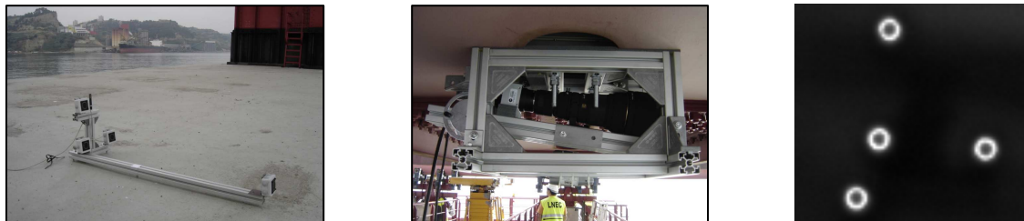
Figures 1 to 3 – Active targets on the south tower foundation (left); digital camera installed in the stiffness girder (center); detail of the image of the targets (right)
