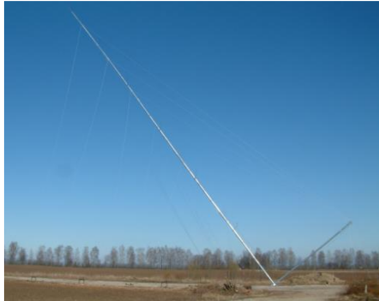
Figure 1. Installation of the 60 m mast with a measuring complex Symphonie (Ainazi site) [2].
