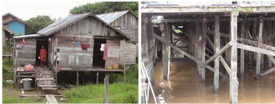
Figure 8. The use of a stage structure for residential buildings on the riverside
