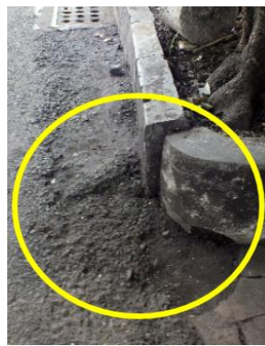
Figure 19. Damage characteristics of score 2 by angiana roots in Laksda Adisucipto street (image source: [23]).
