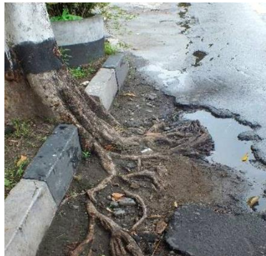
Figure 12. Damage characteristics of score 3 by the root of angšana in Glagahsari street (image source: [23]).
