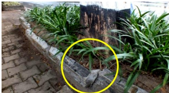
Figure 4. Damage score 2: roots start to slightly appear on the surface and damage the pots (image source: [23]).
