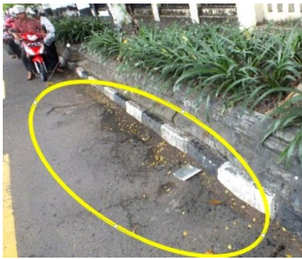
Figure 6. Damage score 3: roots appear to the road surface and make the pots raised (image source: [23]).
