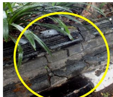
Figure 15. Damage characteristics of score 1 by angana roots in Glagahsari road (image source: [23]).
