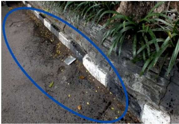
Figure 16. Damage characteristics of score 2 by angiana roots in Glagahsari road (image source: [23]).
