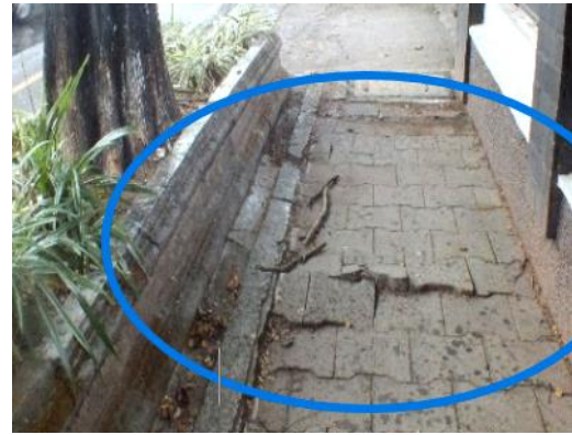
Figure 17. Damage characteristics of score 3 by angiana roots in Glagahsari road (image source: [23]).
