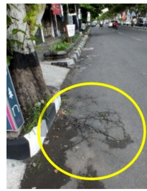
Figure 20. Damage characteristics of score 3 by angiana roots in Laksda Adisucipto road (image source: [23]).
