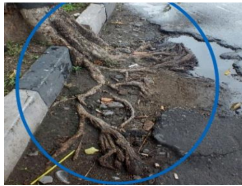
Figure 7. Damage score 3: roots appear to the road surface and cause a bend that can harm road users (image source: [23]).
