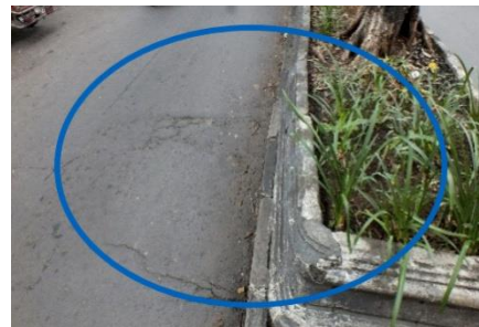
Figure 5. Damage score 2: Roots slightly appear on the surface of the road and cause cracks in the road (image source: [23]).
