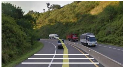
Figure 7. Recommended installation of rumble strips at Km 09 + 300
