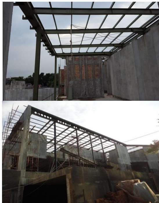
Figure 1. Installation of the roof support.
