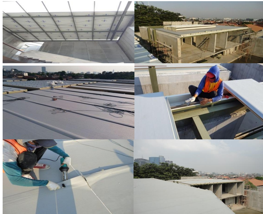
Figure 2. Installation of the insulation panels on project.
