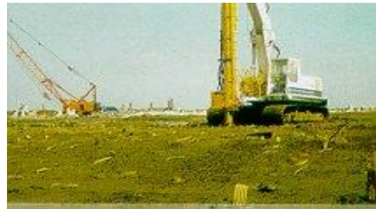
Figure 4. Installation of Fibredrain® at project site
