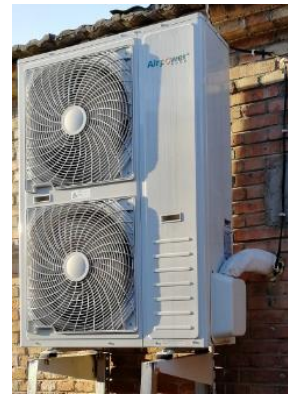
Figure 4. Outdoor part of an ASHP unit at a village in northern China
