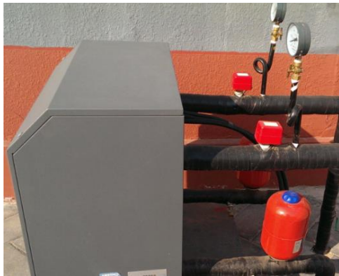
Figure 3. Outdoor part of a GSHP unit at a village in northern China
