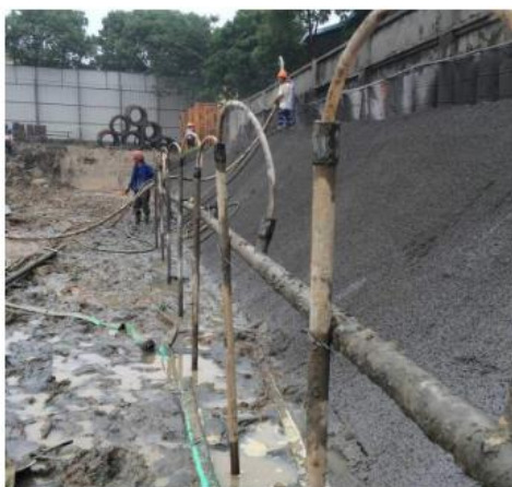
Figure 5. Pipe well dewatering.
