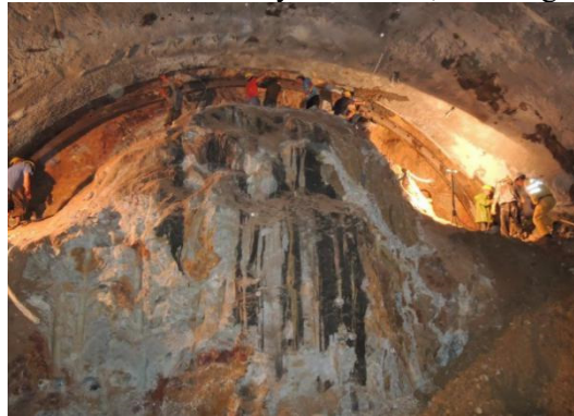
(a) Core pulp consolidation of the tunnel face
