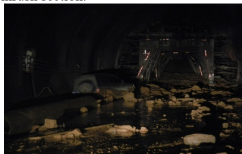
(a) Site of water inrush from left hole mud
