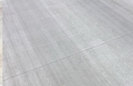
2) Cement surface roughening treatment
