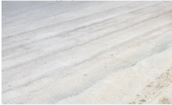
1) Polishing treatment of cement pavement base
