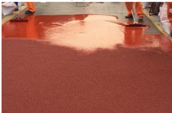
5) Construction of colored aggregate on surface
