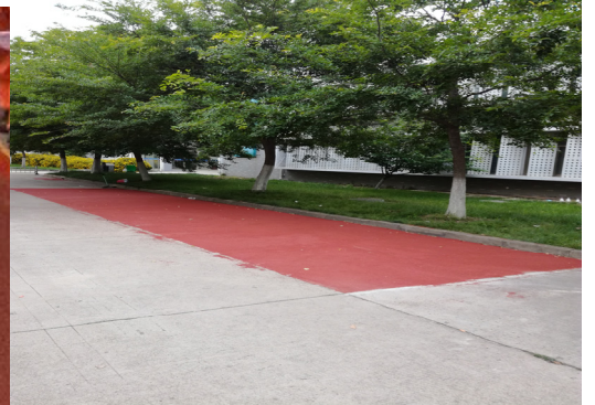
6) Clean surface aggregate after curing and drying
