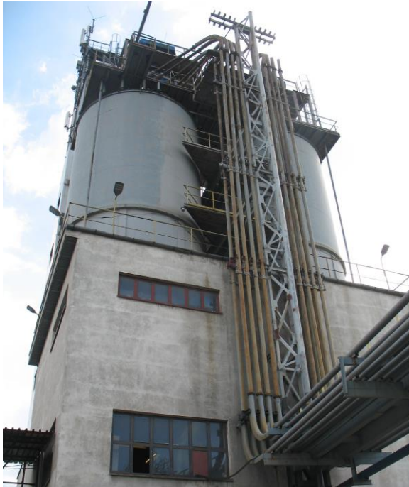
Figure 7. Retention tanks for fly ash.
