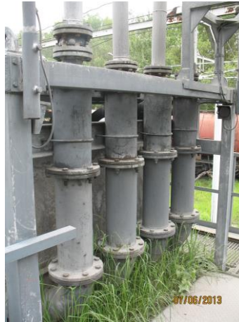
Figure 3. Built-up set of four flow mixers.
