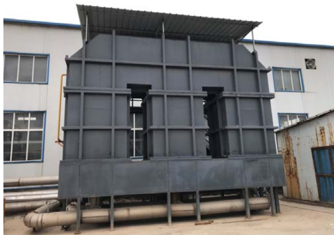
Figure 1. Photographs of three-bed RTO
