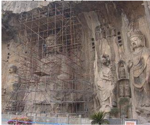
Figure.2 repair and reinforcing site of fengxian temple
