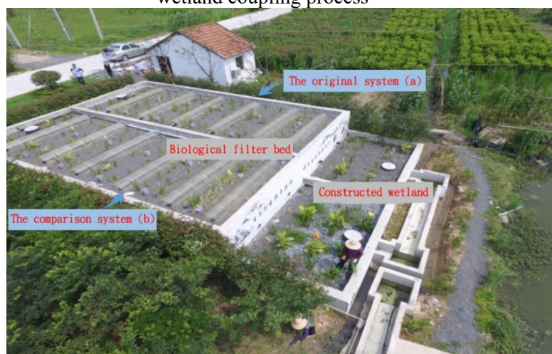
Figure 2-2. The scene of pilot-scale project in Yuhang district of Hangzhou.
