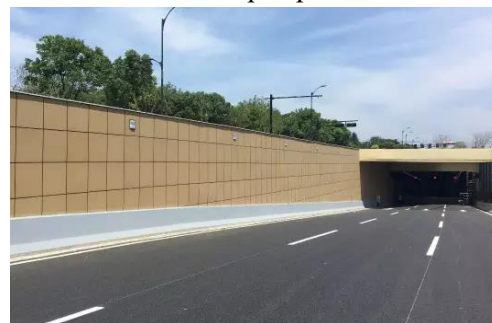
Figure 2. A sound absorbing sandstone plate used in a tunnel
