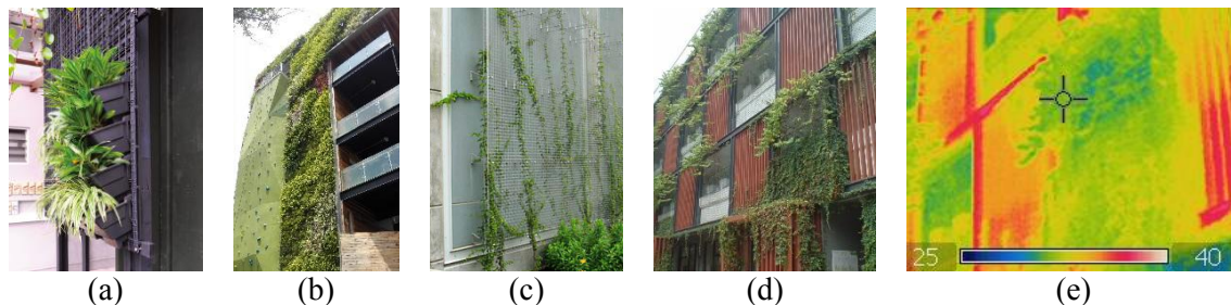
Figure 1. Cases of the LWS and GF (a, b. Detail and façade of LWS; c, d. Detail and façade of GF; e. Thermal image showing that the Temp of the SDs is higher than the GF)
