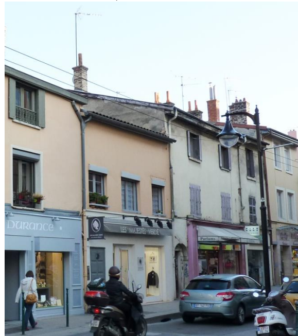
Figure 6. Rammed earth appears under coating in this construction main street of the district ©Craterre
