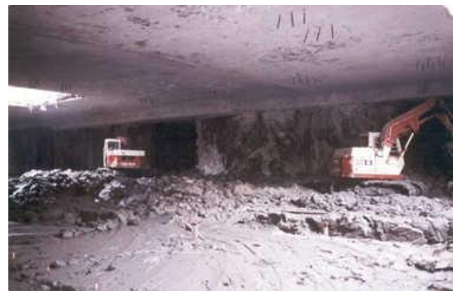
Figure 15. Access openings for excavating in Top-down method.
