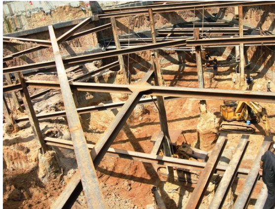
Figure 7. Excavation and bracing steel strut installation in Bottom-up method
