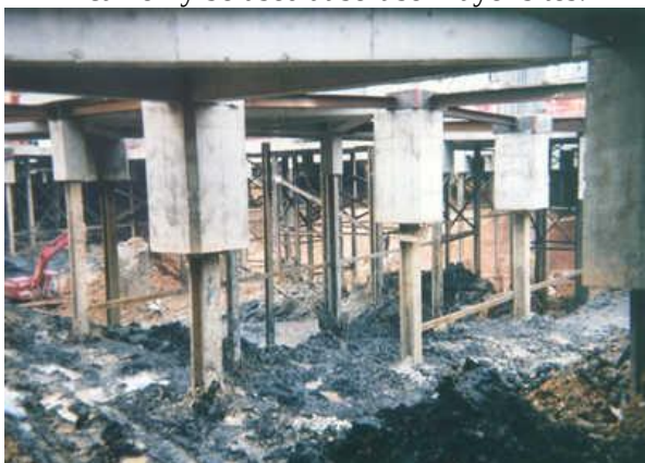
Figure 14. Kingpost (Decking) in Top-down method.
