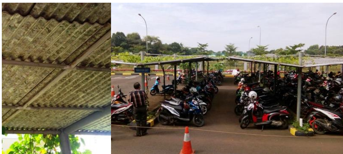
Figure 4. The roof of the parking lot building from waste food packaging.
