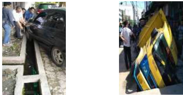
Figure 1. Accident due to open conduit (without cover)
