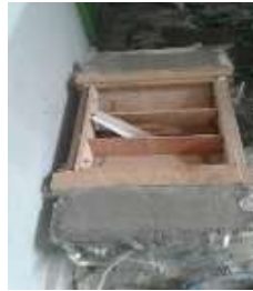
Figure 8. mortar in the mold
