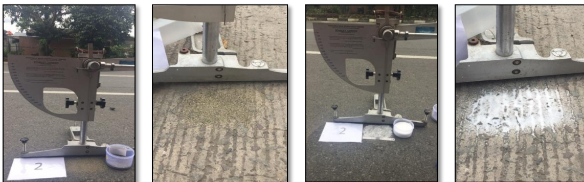
Figure 4. Pavement surfaces affected by sand and salt contaminants
