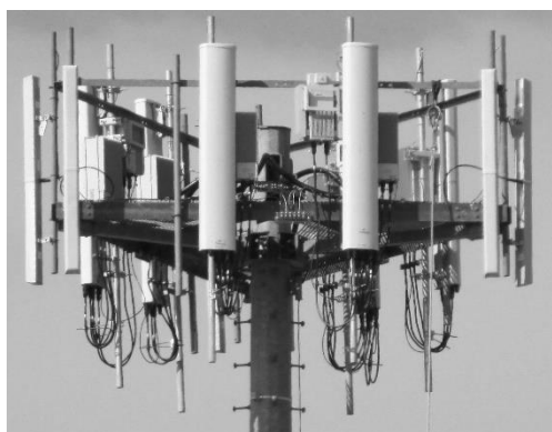
Figure 1 – BTS LTE antenna configuration
