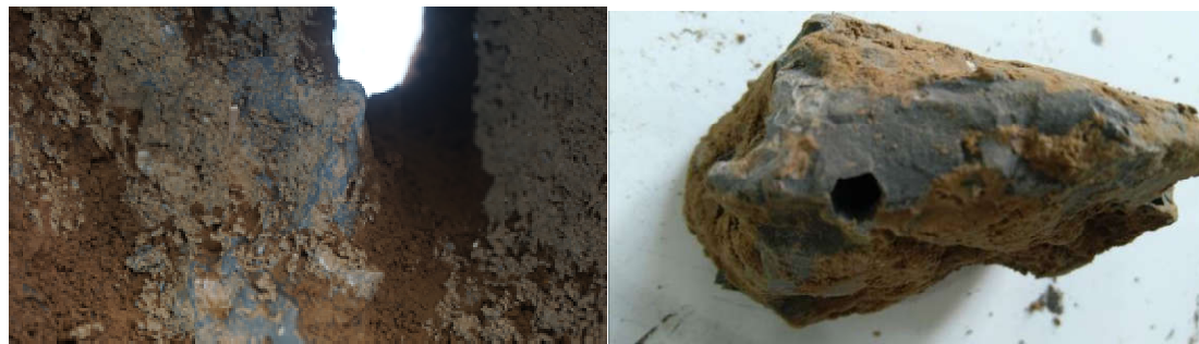
(a) Slurry veins in tunnel
