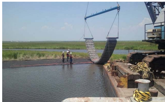
Figure 5. Marine mattresses installed from barge (courtesy Tensar International)
