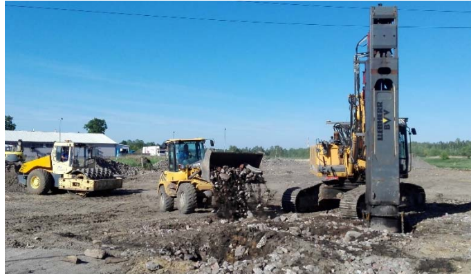
Figure 12. Equipment for Rapid Impulse Compaction (courtesy DABI)
