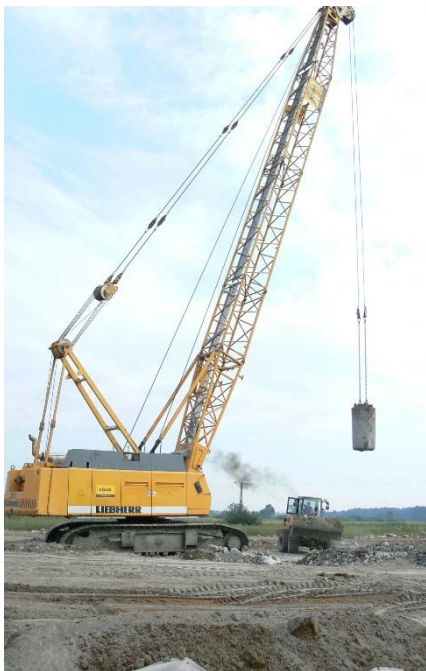
Figure 10. The dynamic replacement - heavy crane with pipe-like rammer
