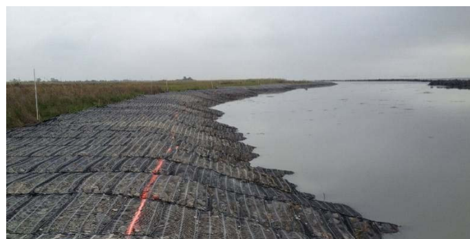
Figure 6. View on completed cost protection Marine mattress (courtesy Tensar International)
