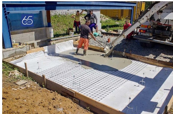
Figure 1. Testing field – concreting of FC reinforced layer
