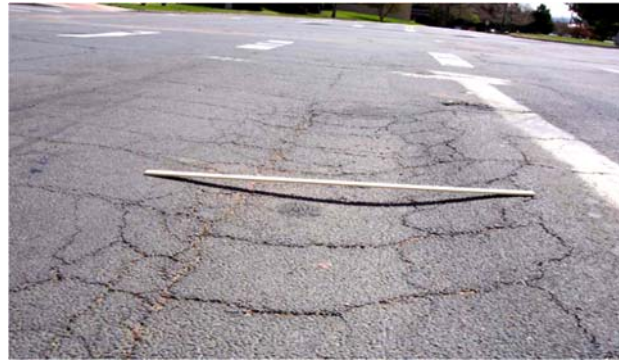
Figure 2. Rutting distress
