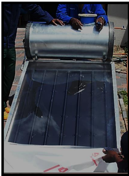
Figure 6. Installing a fixed slope solar collector in a household compound.
