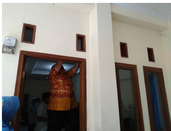
Figure 4. The small ventilations on the upper part of window
