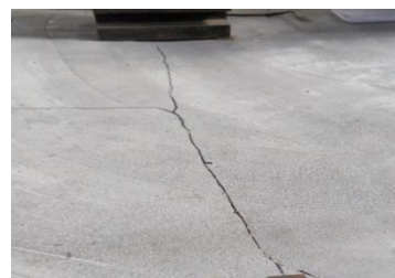
(b) Crack on top surface of concrete
