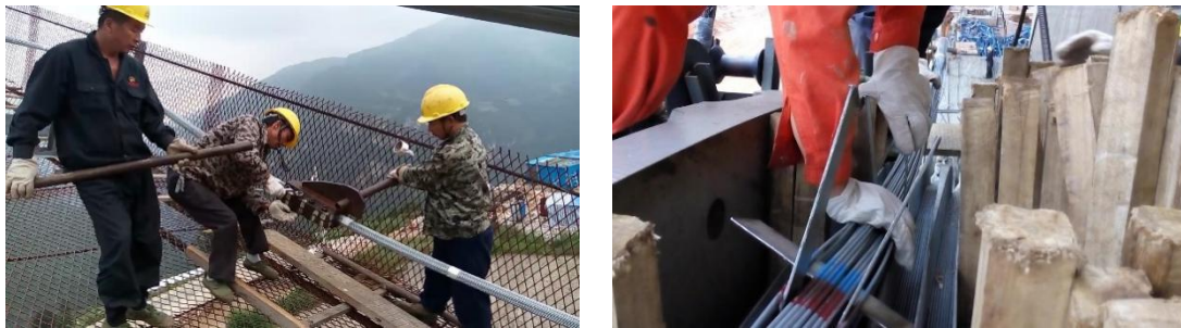
Figure 2 Section Adjustment of Strand
