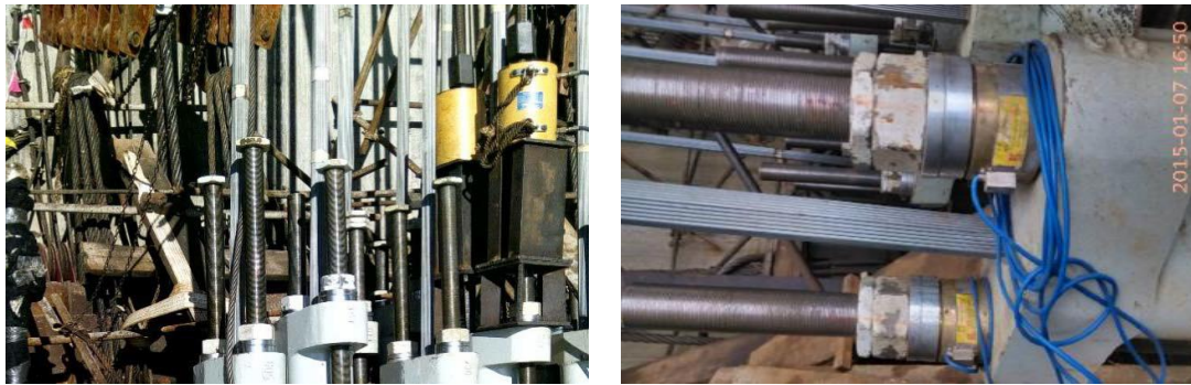
Figure 5 Tension Adjustment of Starnd
