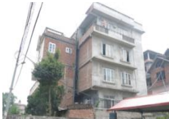
Fig.11 Collision damage to adjacent structures
