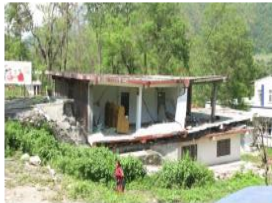
Fig.12 Collision damage between self-built reinforced concrete frame structure and highway roadbed
