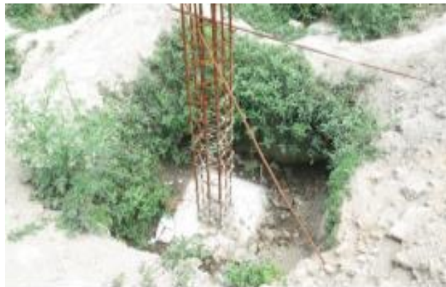
Fig. 3 Reinforcement of frame column
