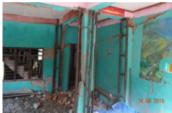
Fig.9 Destruction in the middle of the bottom frame columns
