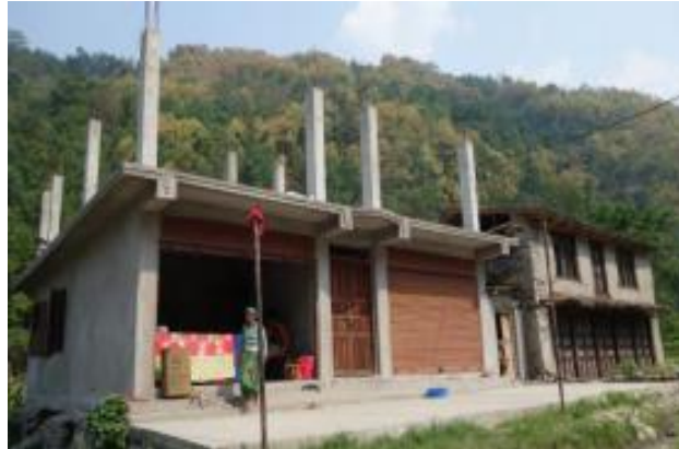
Fig.2 Reserved reinforced concrete column and steel cage on the top floor
