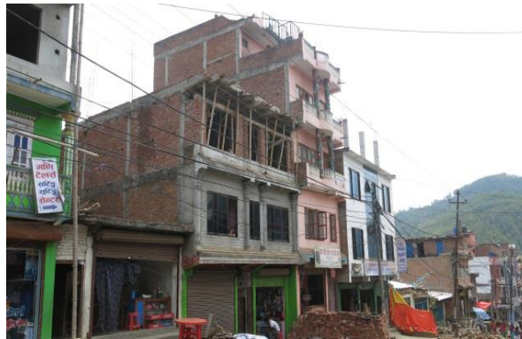
Fig.1 Overall picture of self-built reinforced concrete frame structure
