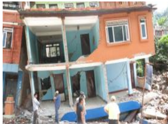
Fig.10 Collapse of the self-built reinforced concrete frame structure
