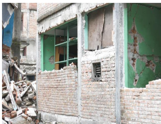
Fig.7 Destruction of infilled walls in the region of IX degrees
