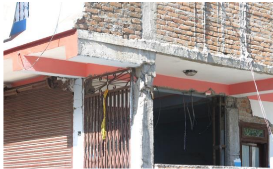
Fig.8 Destruction of the top of the underlying columns in the region of VIII degrees
