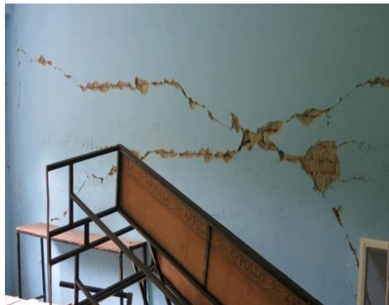
Fig.6 Destruction of infilled walls in the region of VIII degrees
