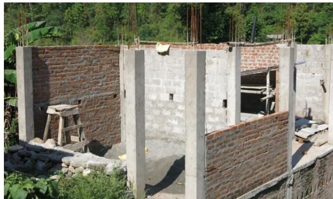
Fig.4 Structural Rachel measures between infilled walls and frame columns are not set
