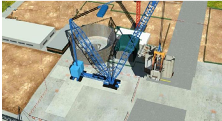
Figure1. Simulation of the large-scale lifting in a NPP project
