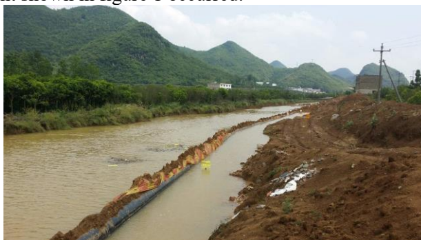
Fig.1 Site photo of floating pipeline
