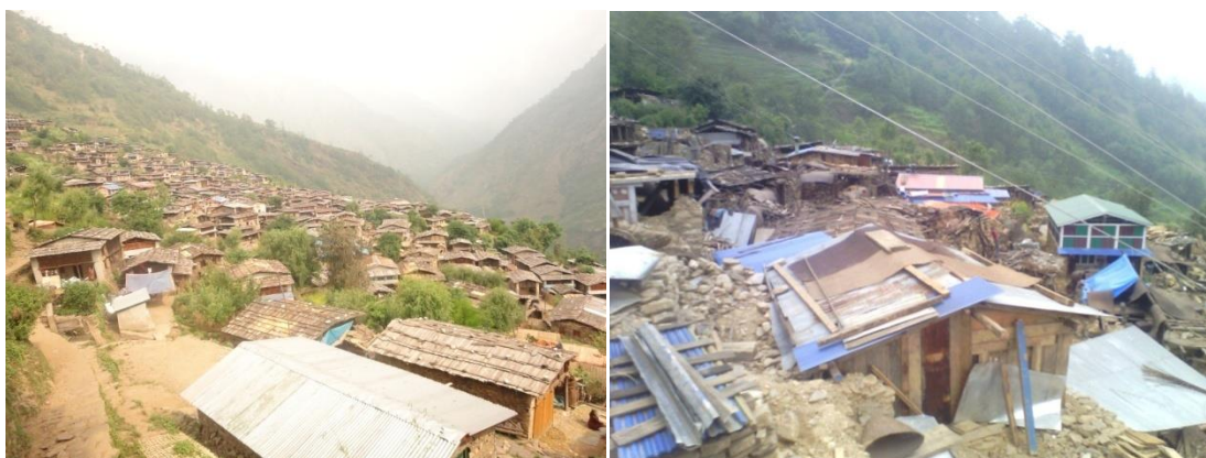
Figure 2. Laprak in Gorkha district before (left) and after earthquake (right)
