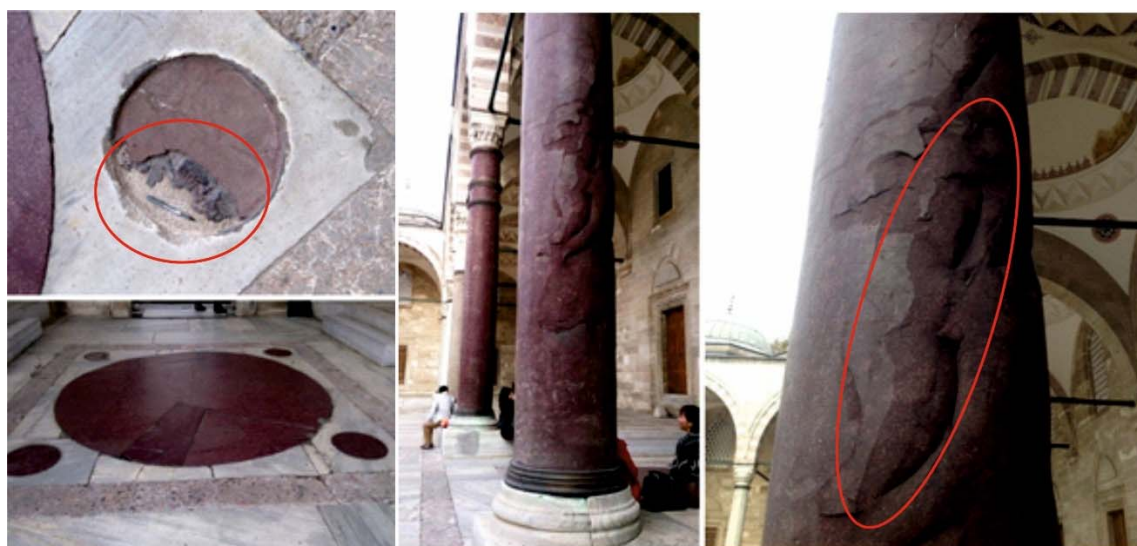
Figure 7. Cracking and loss occur with freeze-thaw effect on the porphyry column and floor
