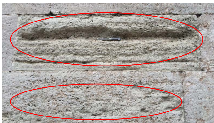
Figure 6. The view of karst in Kufeki Stone
