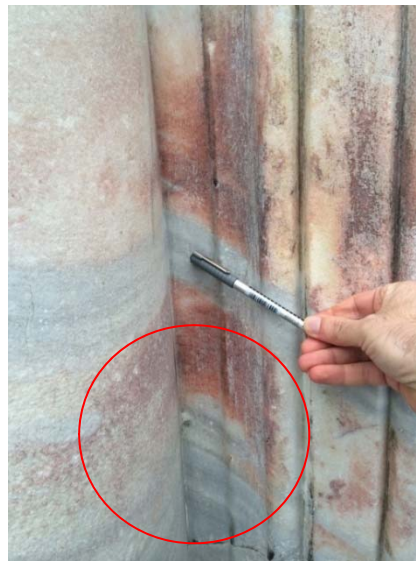
Figure 10. The colour change due to composition of marble
