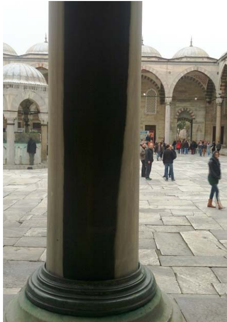
Figure 8. The view of black crust on Marmara Marble
