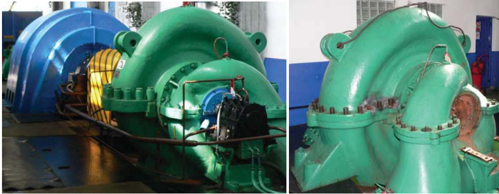
Fig. 1 Unit installed into the pumped storage power plant (left) and the double flux pump (right)
