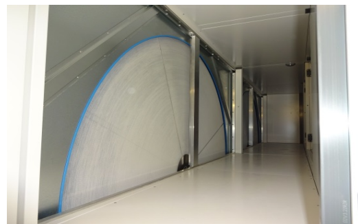
Figure 4: Rotation heat exchanger
