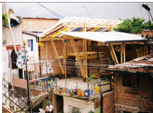
Figure 14. Taller Tropical, two-story bamboo structure located on the first floor
