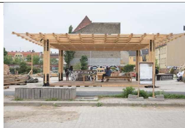
Figure 10. Infozentrale, raw construction, timber beam grillage, fixed columns
