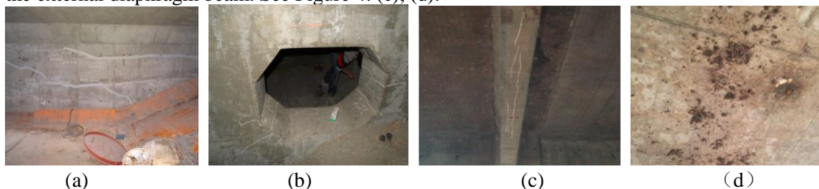
Figure 4. Typical crack diagram of the box girder diaphragm.
