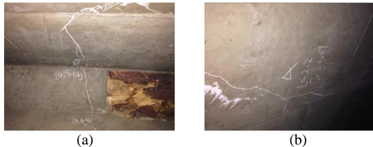
Figure 3. Typical crack diagram at the bottom of the box girder roof.
