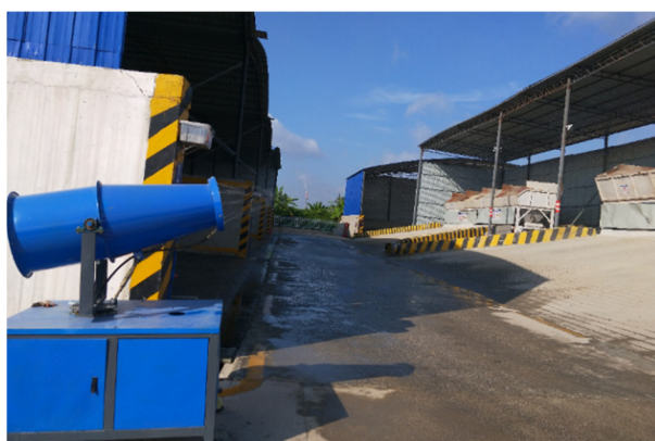
Fig. 1 Dust removal by water spraying in the excavation process
